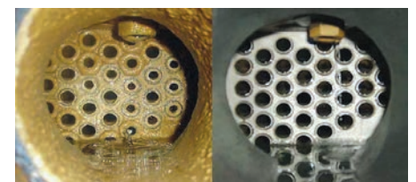
Actual results on a chiller using Dynamic Descaler
