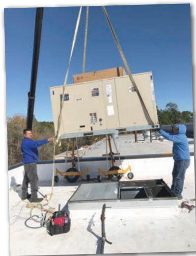
New Allied Z Series unit being lowered onto existing curb
